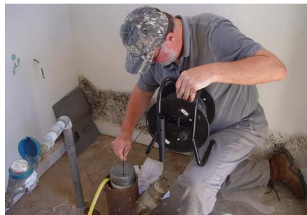
Rene Barker using coaxial cable device to measure depth to groundwater in water-supply well at Fort Davis National Historic Site, April 2008.
