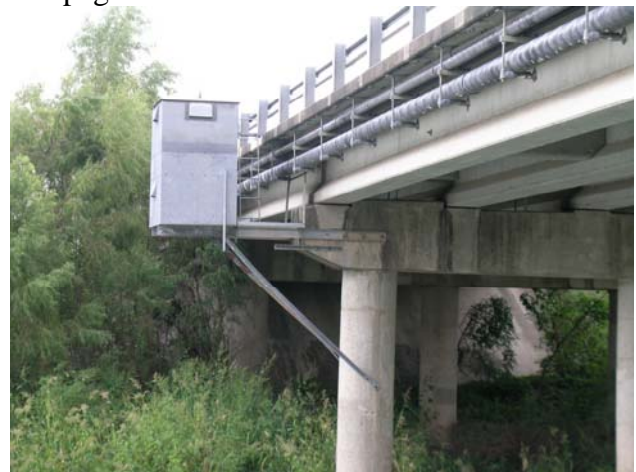
Water quality monitoring station in support of TCEQ's SEP program.
