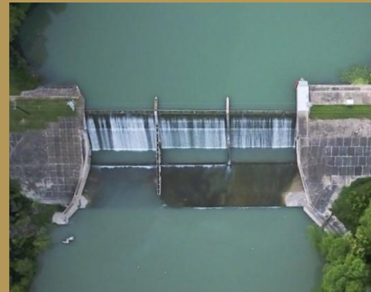
Figure 2: Aerial view of Lake Dunlap dam
