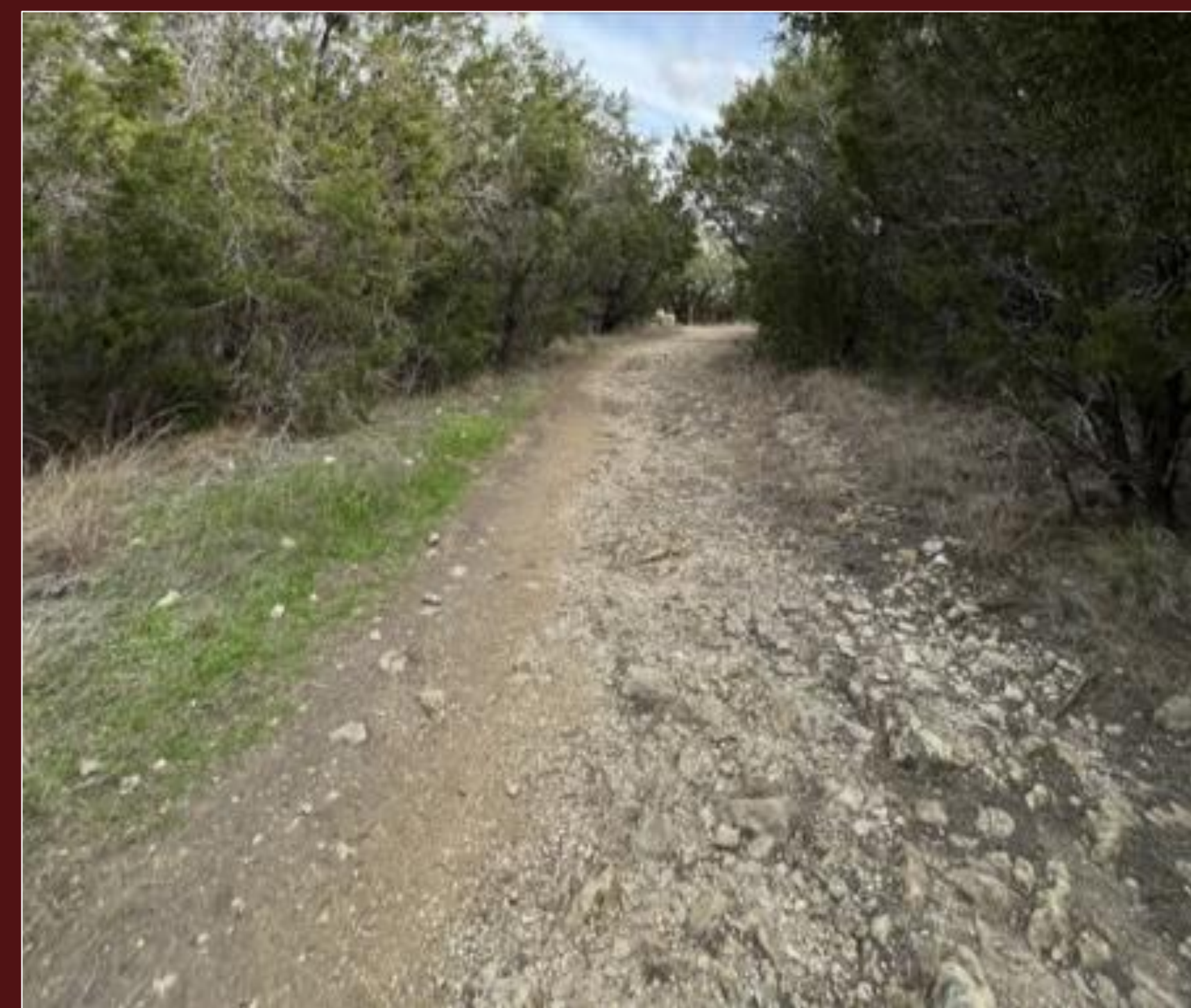
The 140-foot section of Spring Lake Trail
