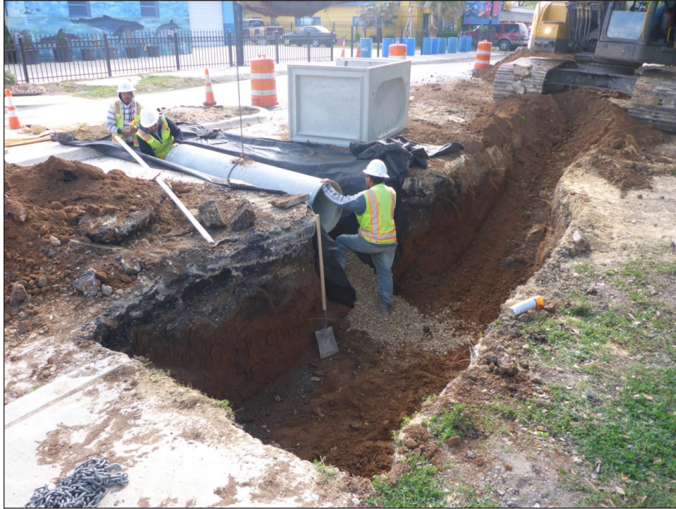
Figure 8. Storm drainage pipe trench, facing east.
