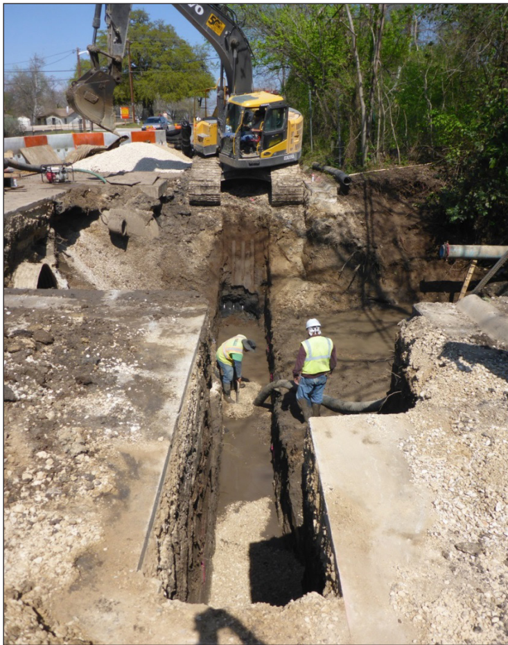
Figure 6. Water main trench, facing northeast.
