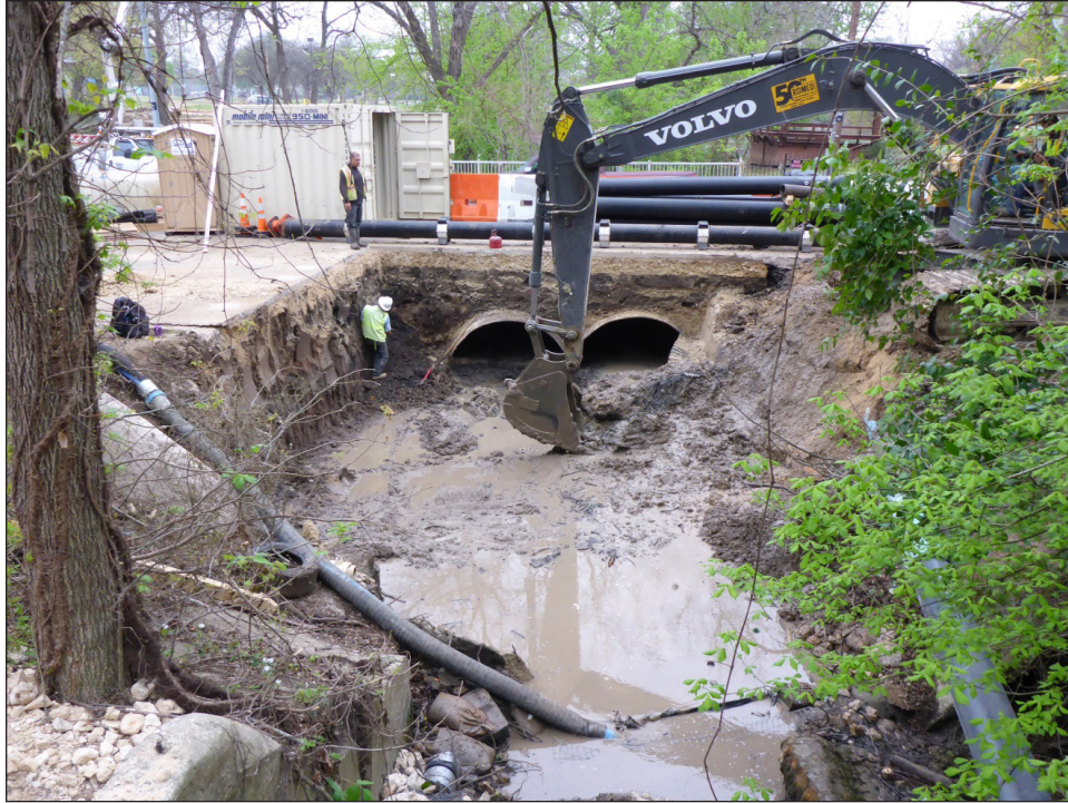
Figure 7. Outflow reconstruction culvert trench (excavation block), facing northwest.
