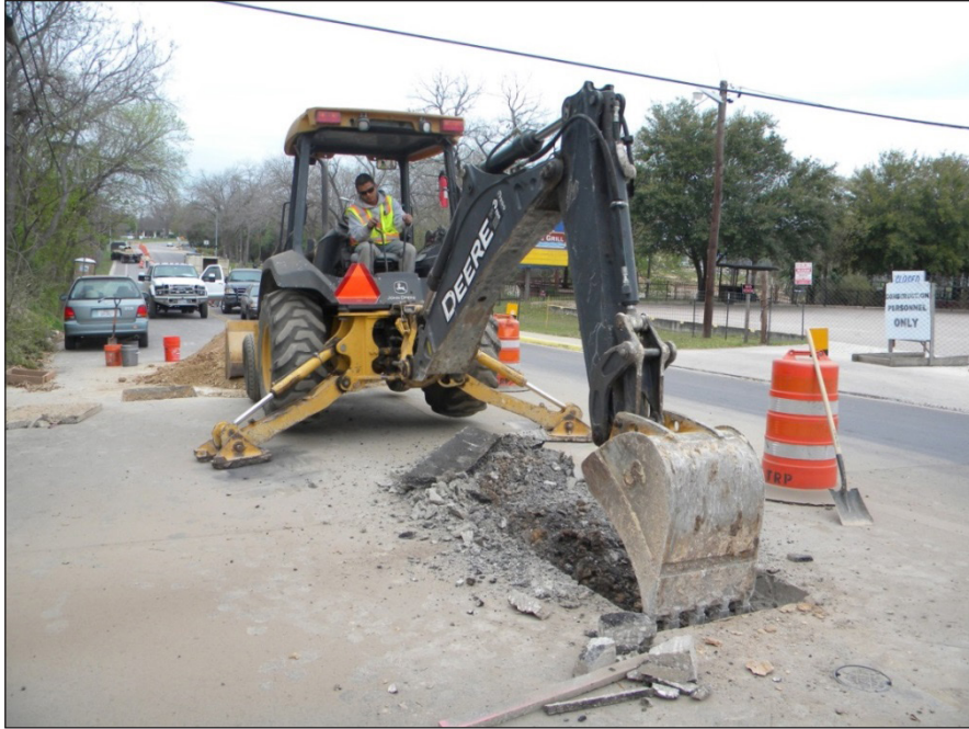
Figure 5. Water main locate and installation trench.
