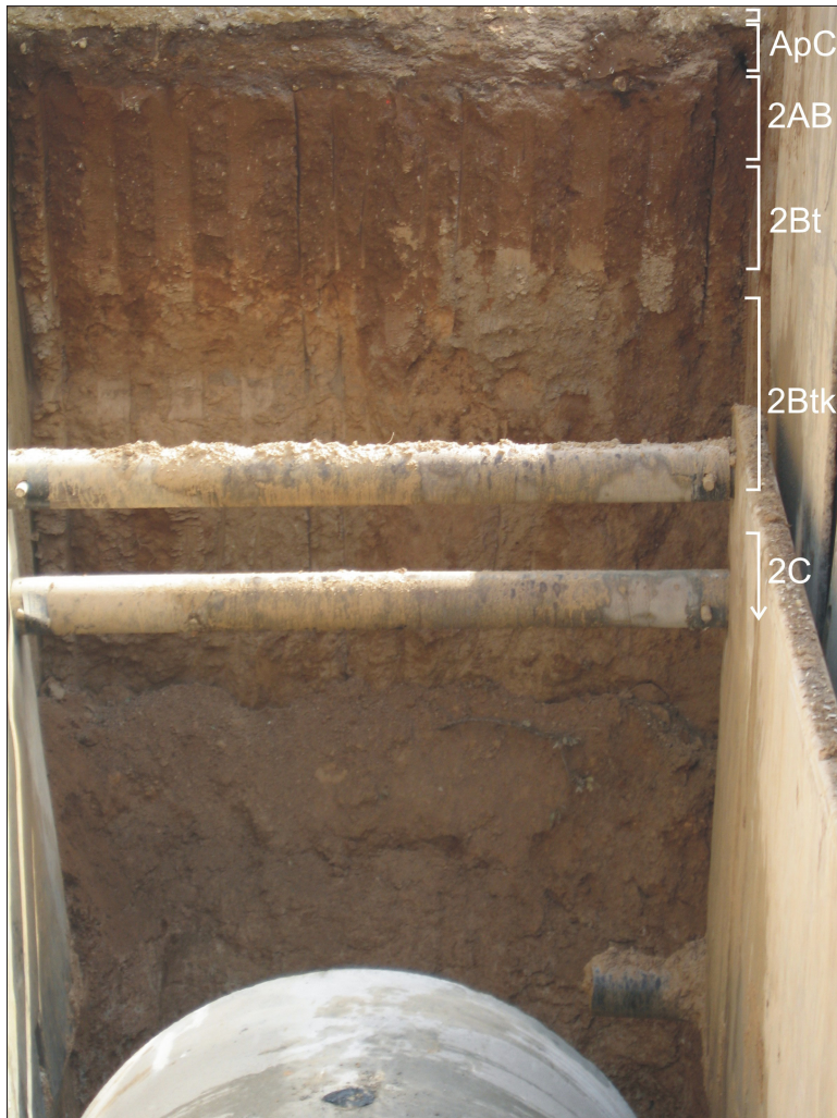
Figure 7. Trench profile exposure, west of Cheatham Street.
