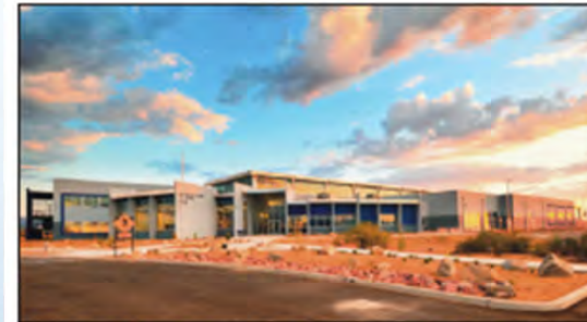
Orenco's AdvanTex ® Wastewater Treatment System was installed at the Andriada Politechnico Palano High school campus near Tucson. (Story on back)
