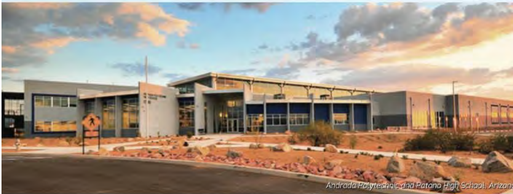
Andrada Polytechnic and Patano High School, Arizona.
