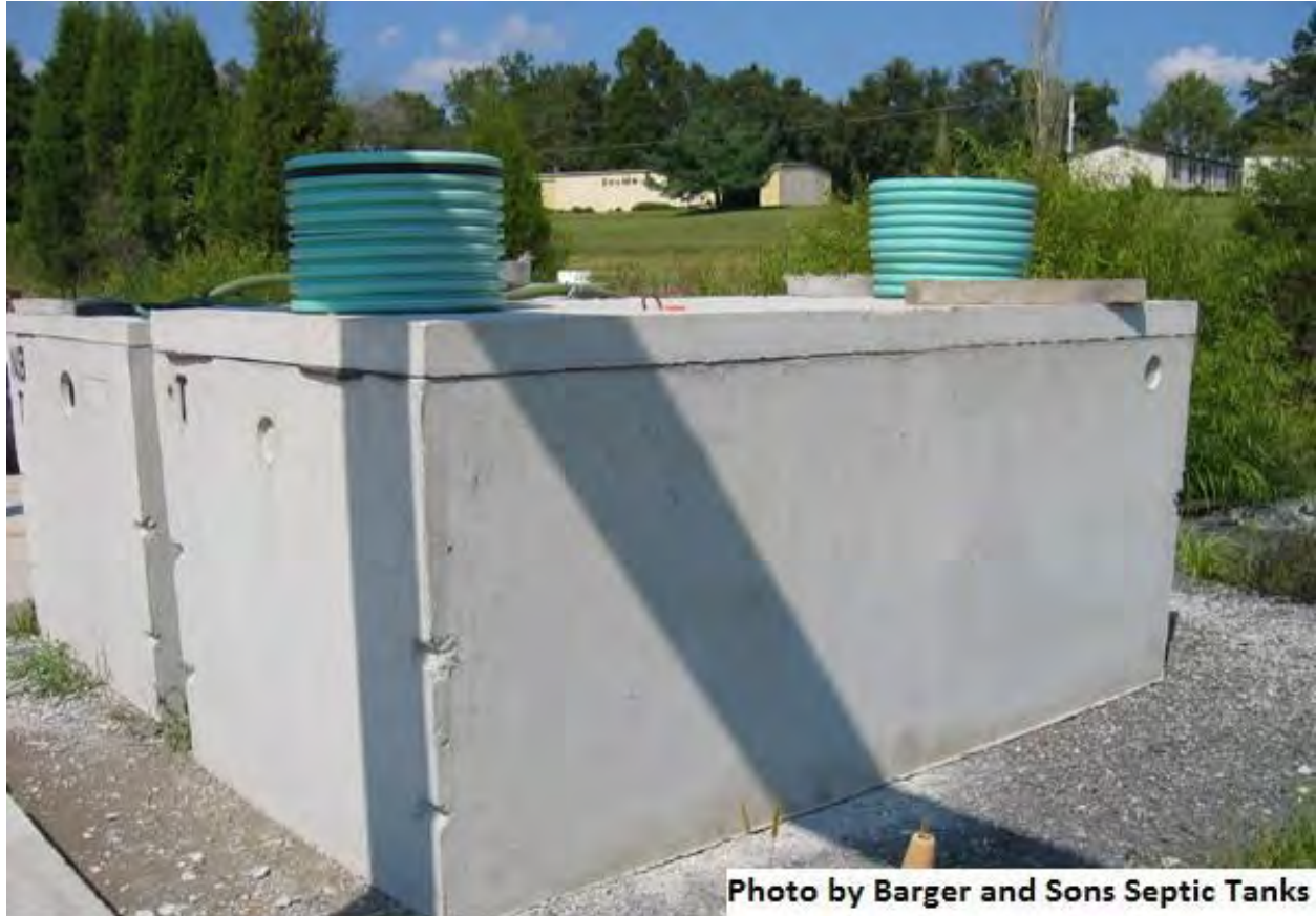
Photo 10: Primary tank being water-tested.
