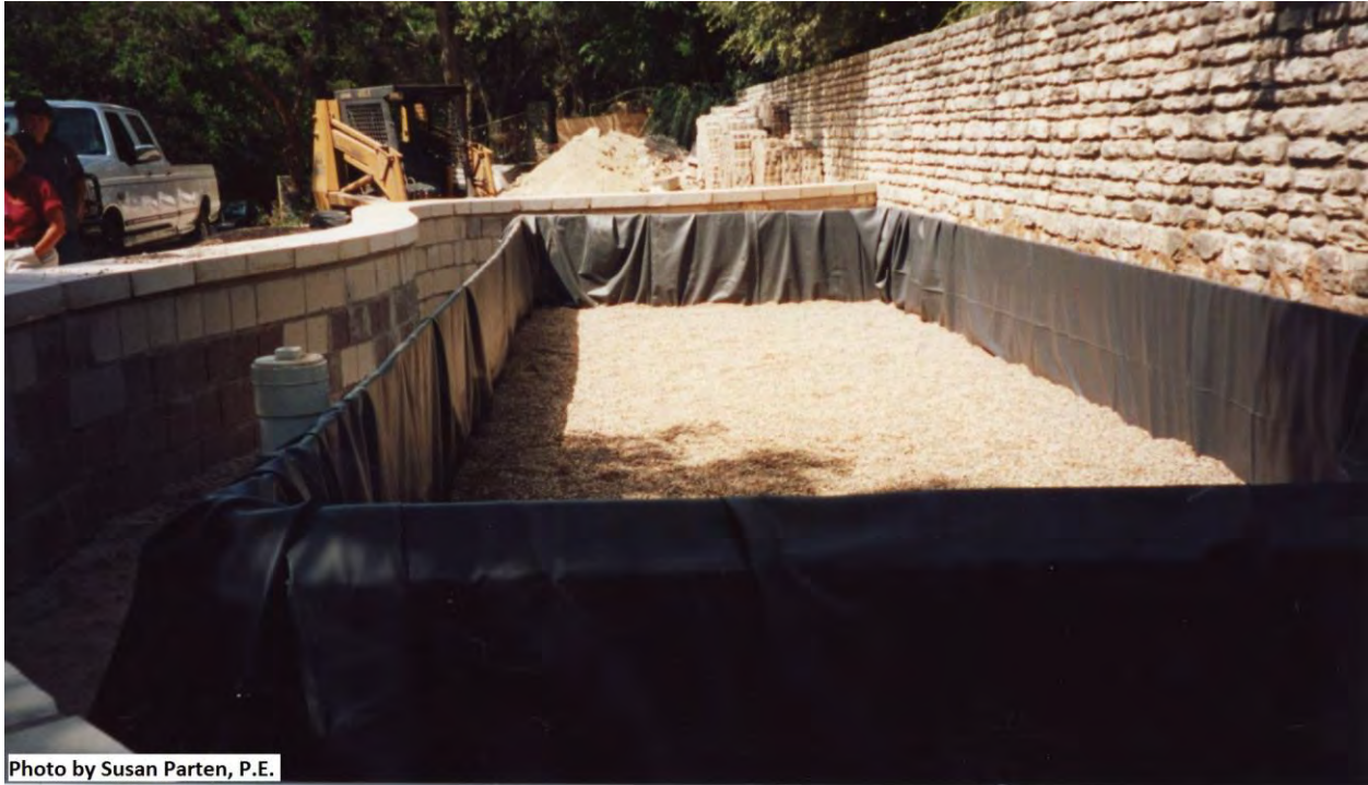
Photo 5: Intermittent sand filter under construction inside stone landscaping wall.
