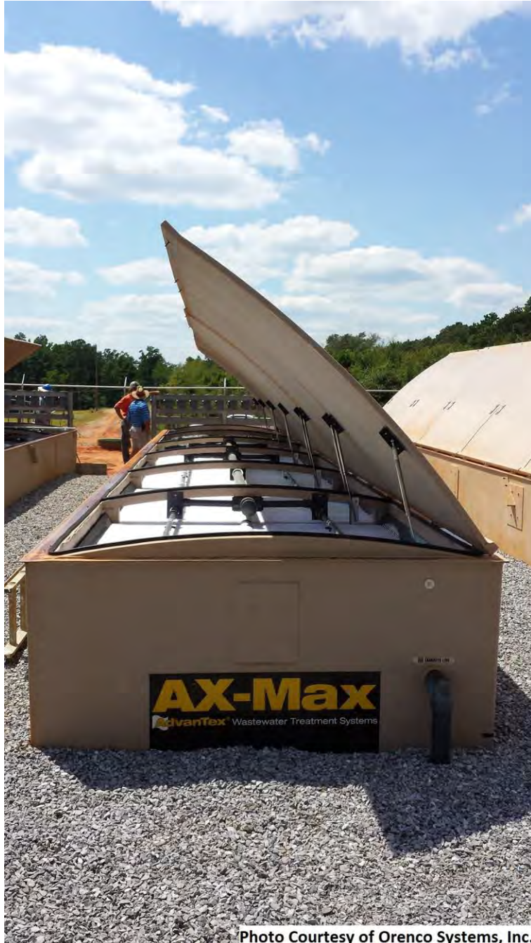
Photo 17: AX-MAX treatment units, opened.
