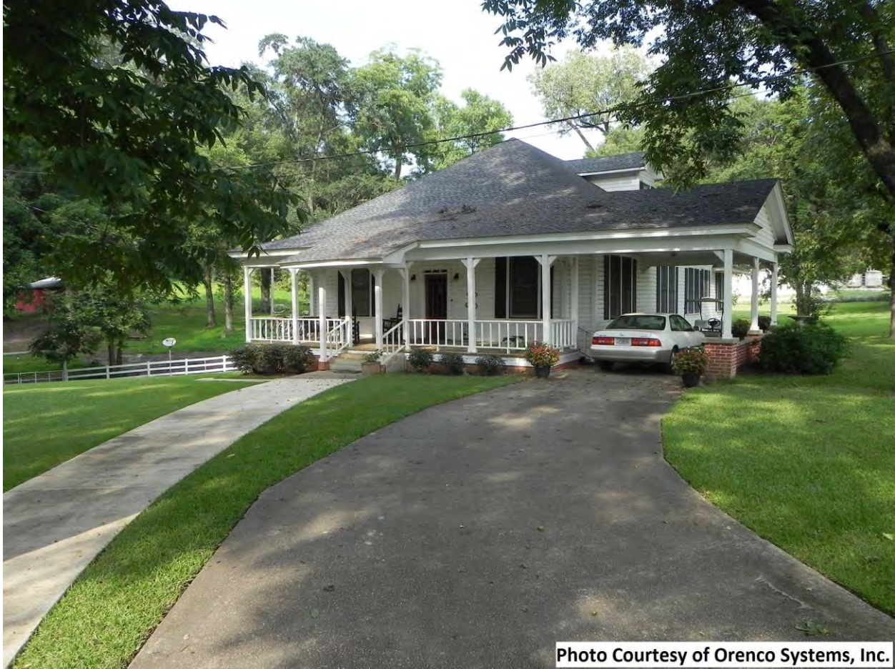
Photo 14: Residence in Fulton, AL.
