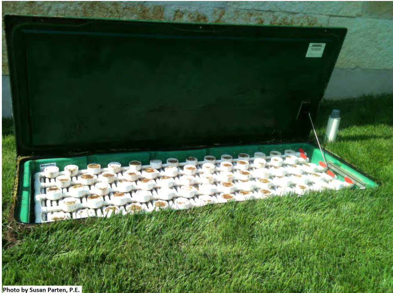
Photo 2: Recirculating media filter unit opened for checks/testing.
