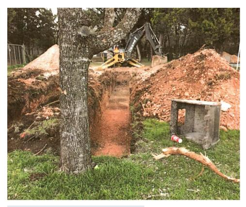
Figure 6. Conventional Trench and Spoil Pile
