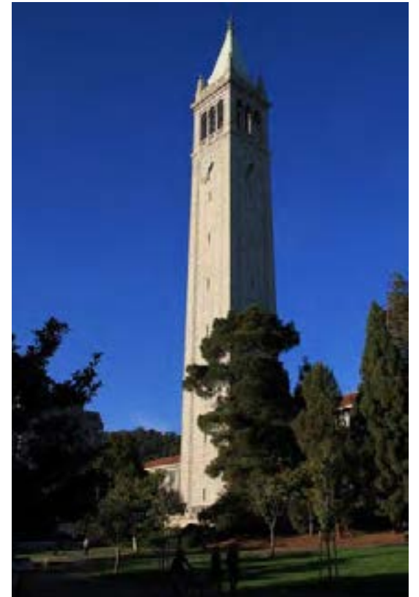
Sather Tower - University of California at Berkeley
