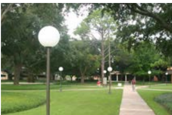
Existing conditions: lighting
