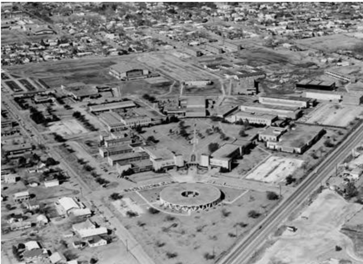
An early aerial view of the campus
