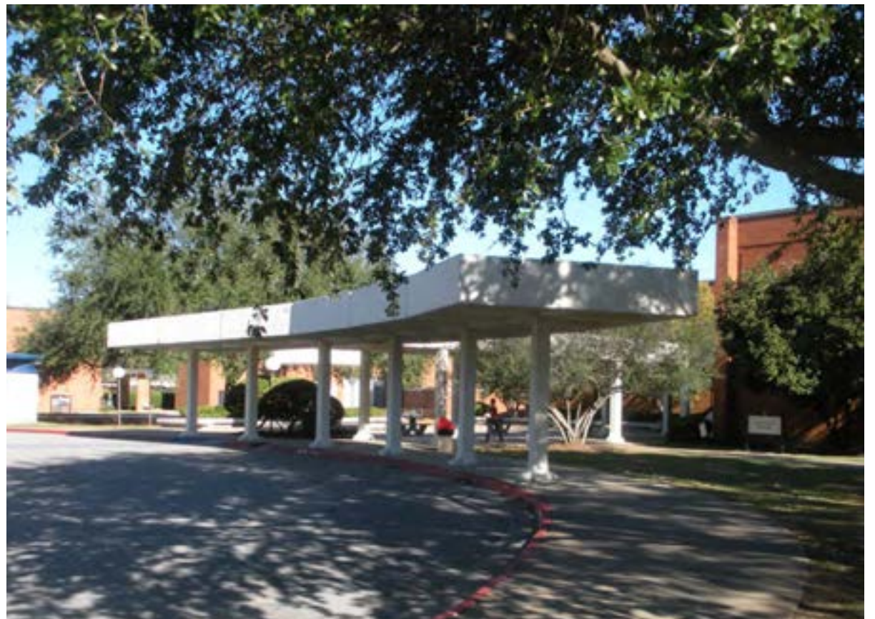
Existing covered walkway west of Setzer Center
