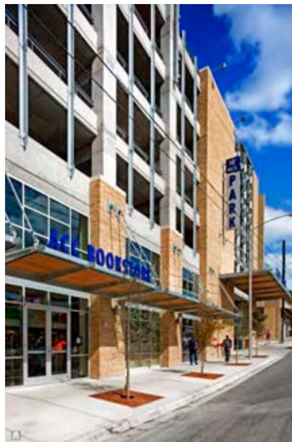
Mixed-use parking garage . Austin Community College
