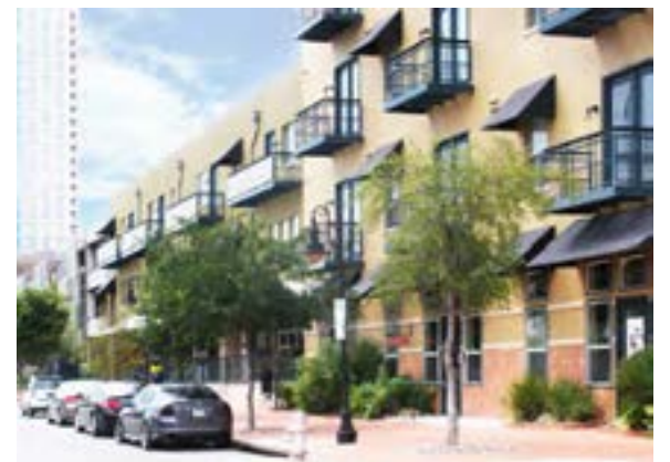
Austin TX - 5th Street, facing east
