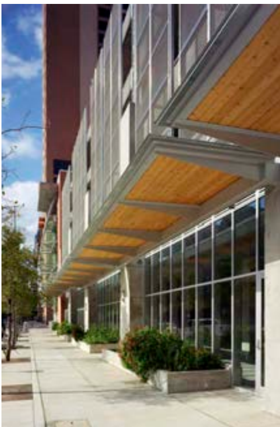
Austin Convention Center Parking Garage with mixed-use
