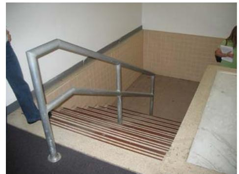
Handrails/Guardrails Not ADA Compliant
