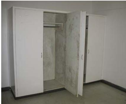
*Poor Indoor Air Quality and Mold Evident Throughout Unoccupied Portion of Building*
