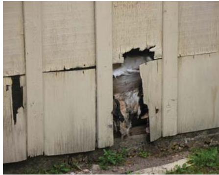
Exterior Wall Rotted and in Very Poor Condition
