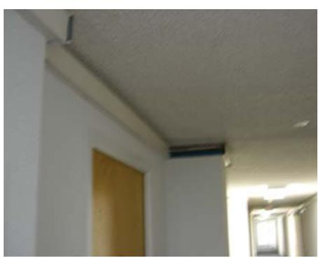
*Electrical Run in Raceway*
