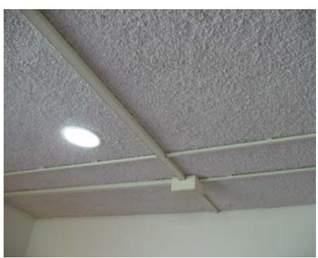
*Electrical Run in Surface-Mounted Conduits*
