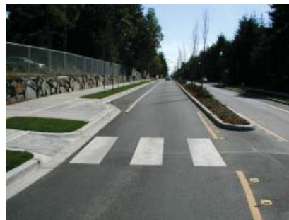
Bump-outs provide a permanent solution to slow vehicular traffic at deliberate pedestrian crossings. Image: www.peopleforbikes.org /Dan Burden
