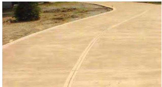
*Standard colored concrete: 3000 psi min. concrete paving with medium broom finish, Scofield Color "Autumn Beige" integral additive.*
