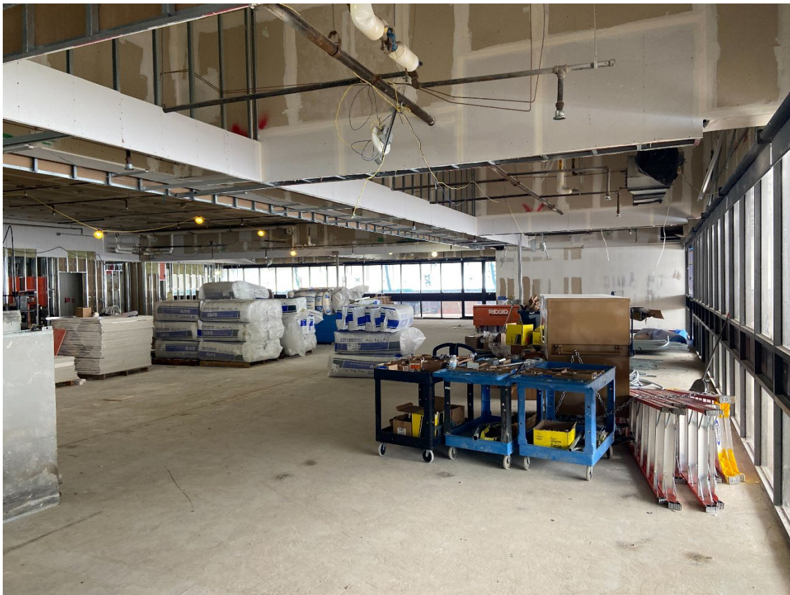
New Interior Drywall Installation Underway
