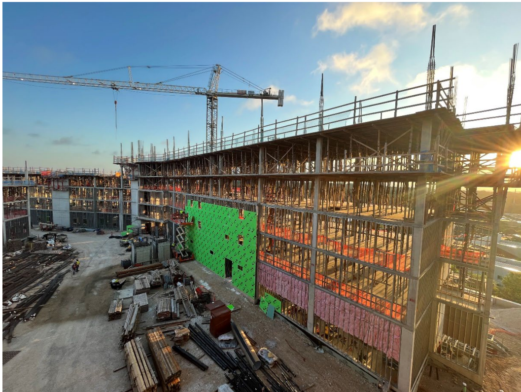
Exterior Framing - North Tower
