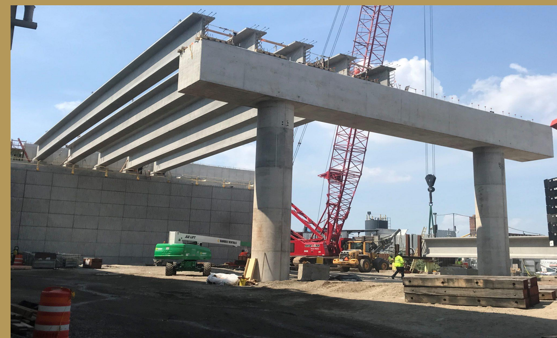
The prestressed concrete I-girder (T-62)
