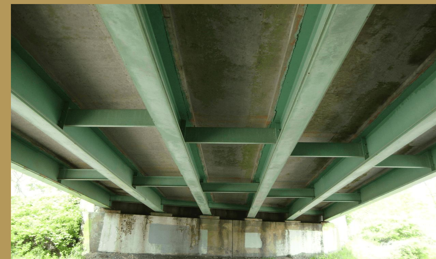
The Steel I-girder beam (Rolled).
