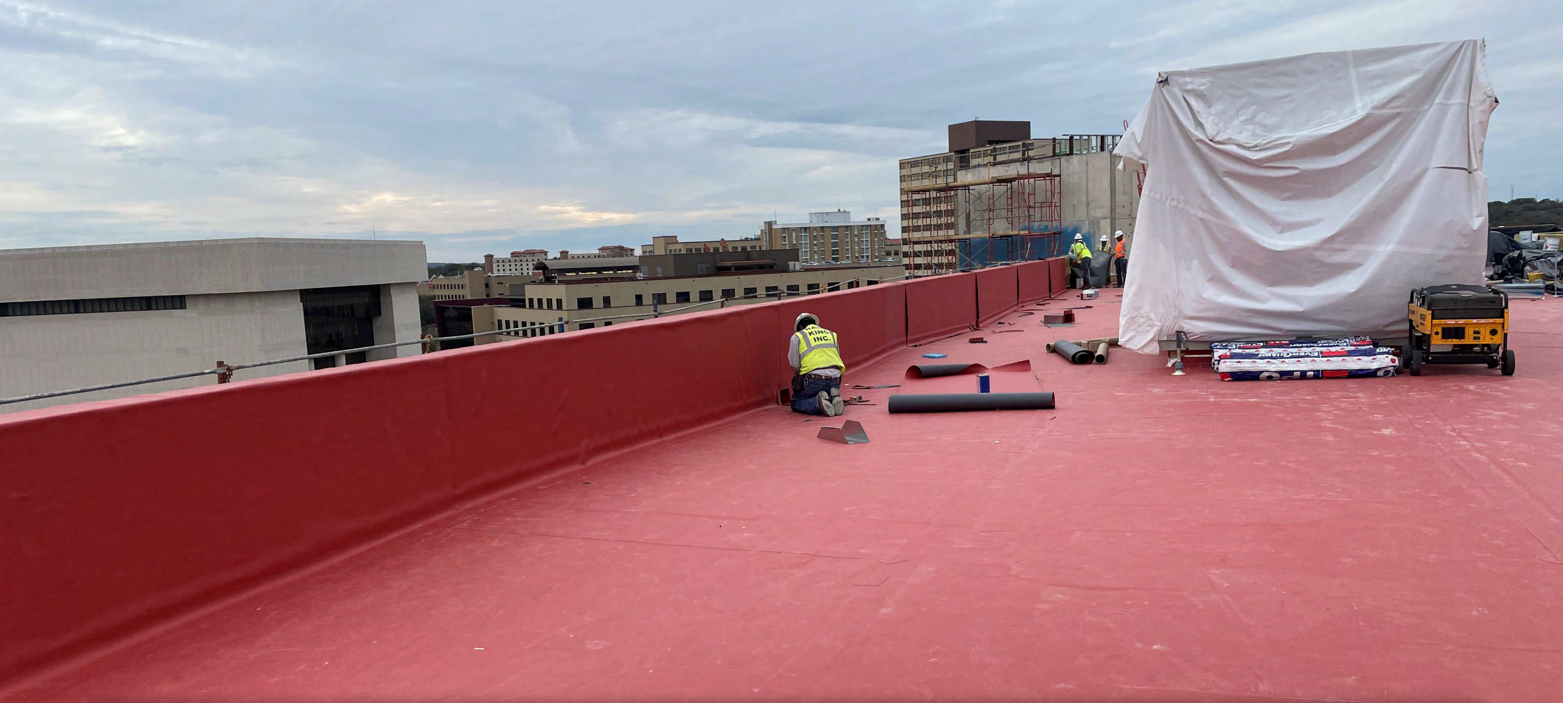
Roofing Installation (Alamito)
