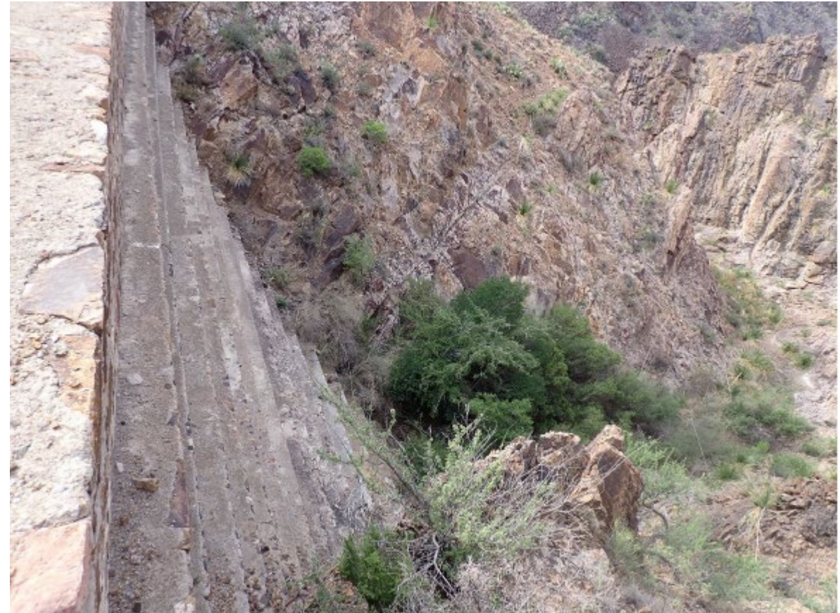
Downstream view from top of Dam
