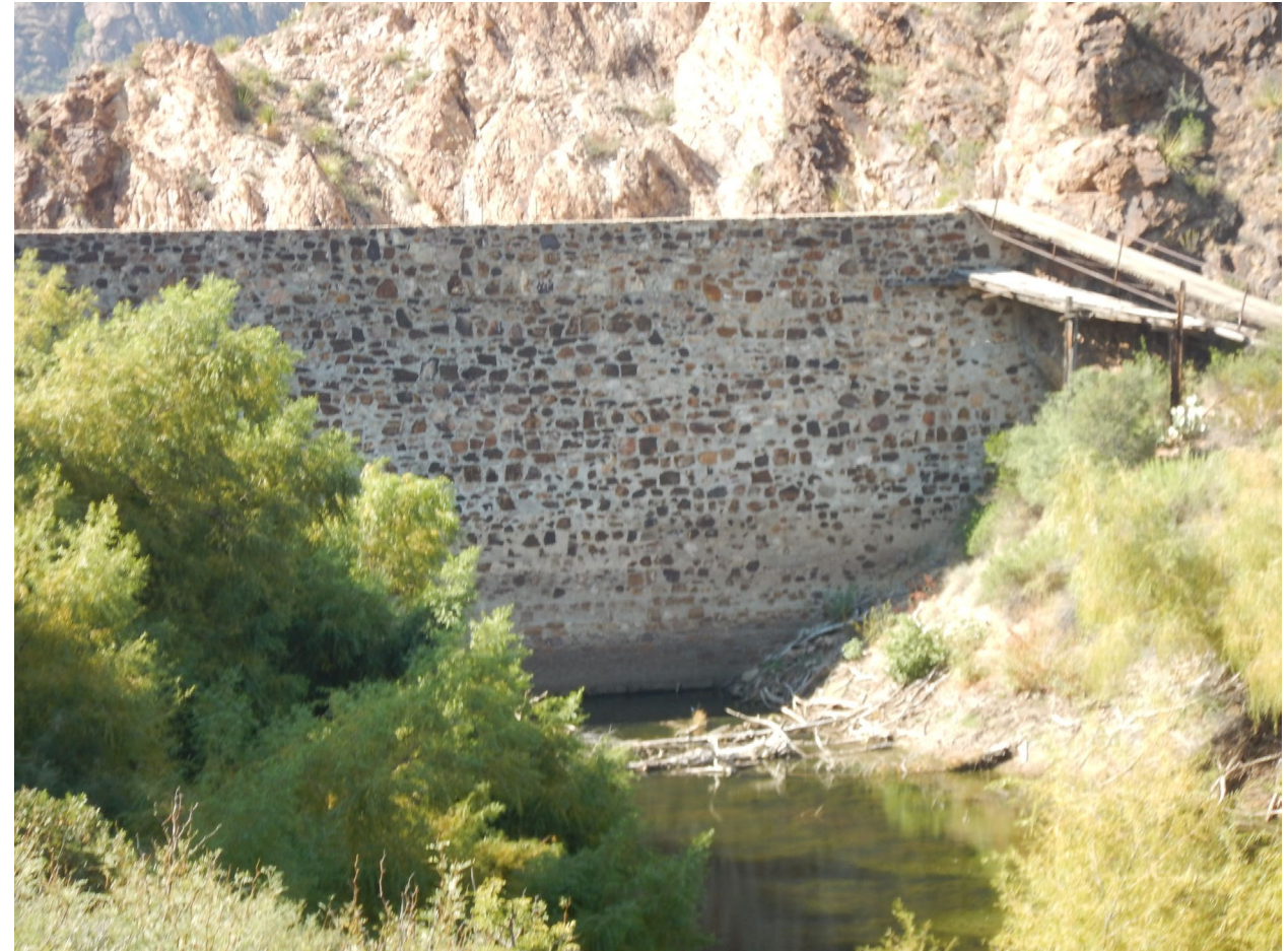
Close-up view with access bridge to the right
