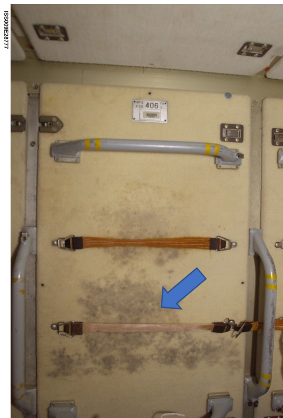
FIG 3 Fungal contamination of a noise mitigation panel in the ISS Zarya module where exercise and hygiene clothes were hung to dry. The arrow points to areas discolored by fungus. (Image from NASA, photo iss009E28777.)
