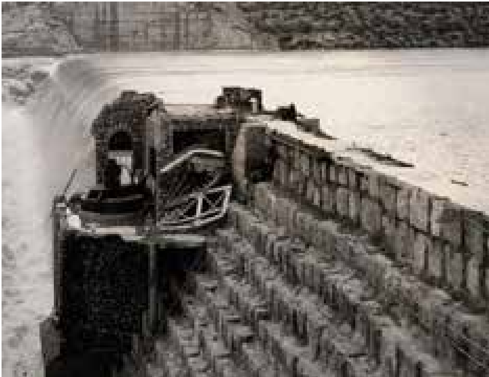
Figure 11. Devils Lake Dam (National Park Service [NPS], n.d.)
