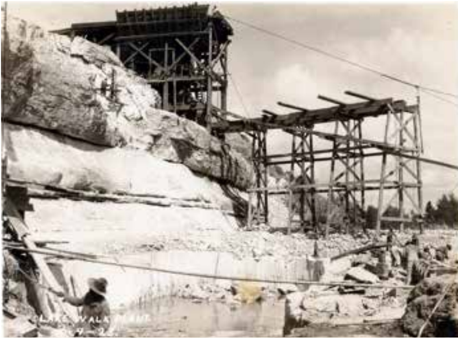
Figure 12. Lake Walk Plant Construction (NPS, n.d.)
