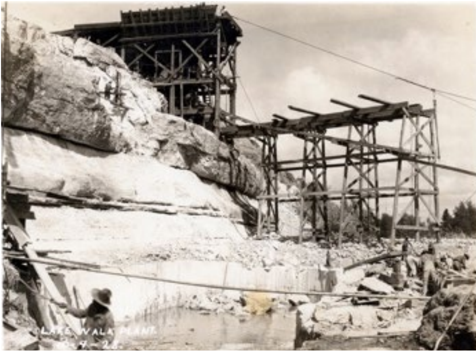
Figure 12. Lake Walk Plant Construction (NPS, n.d.)
