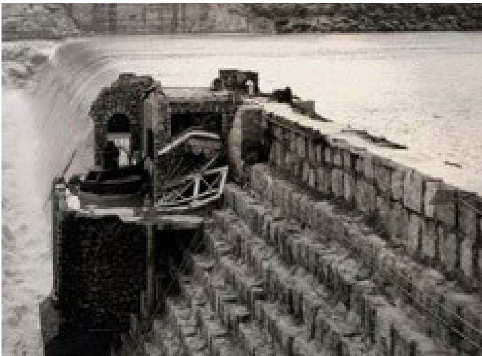
Figure 11. Devils Lake Dam (National Park Service [NPS], n.d.).
