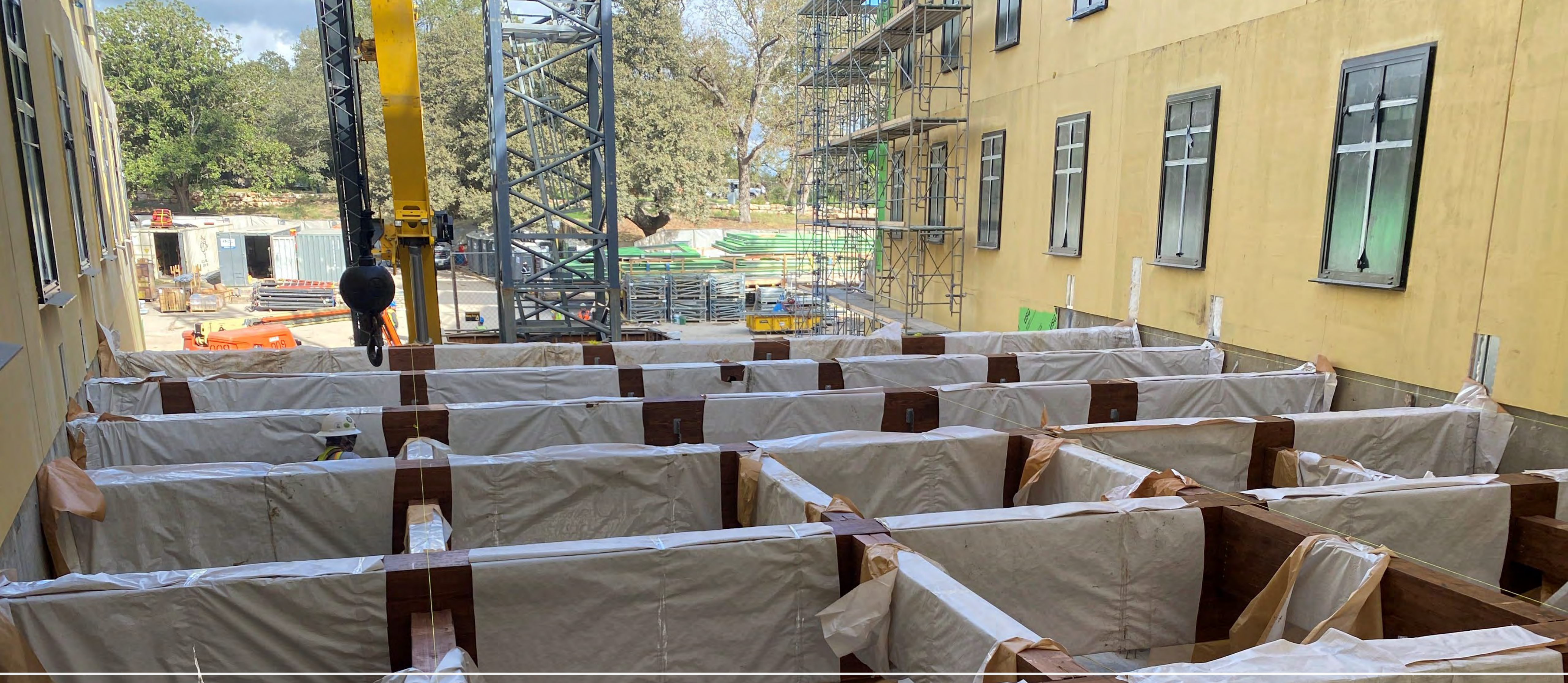
Level 1 – Wood Beams at Entry
