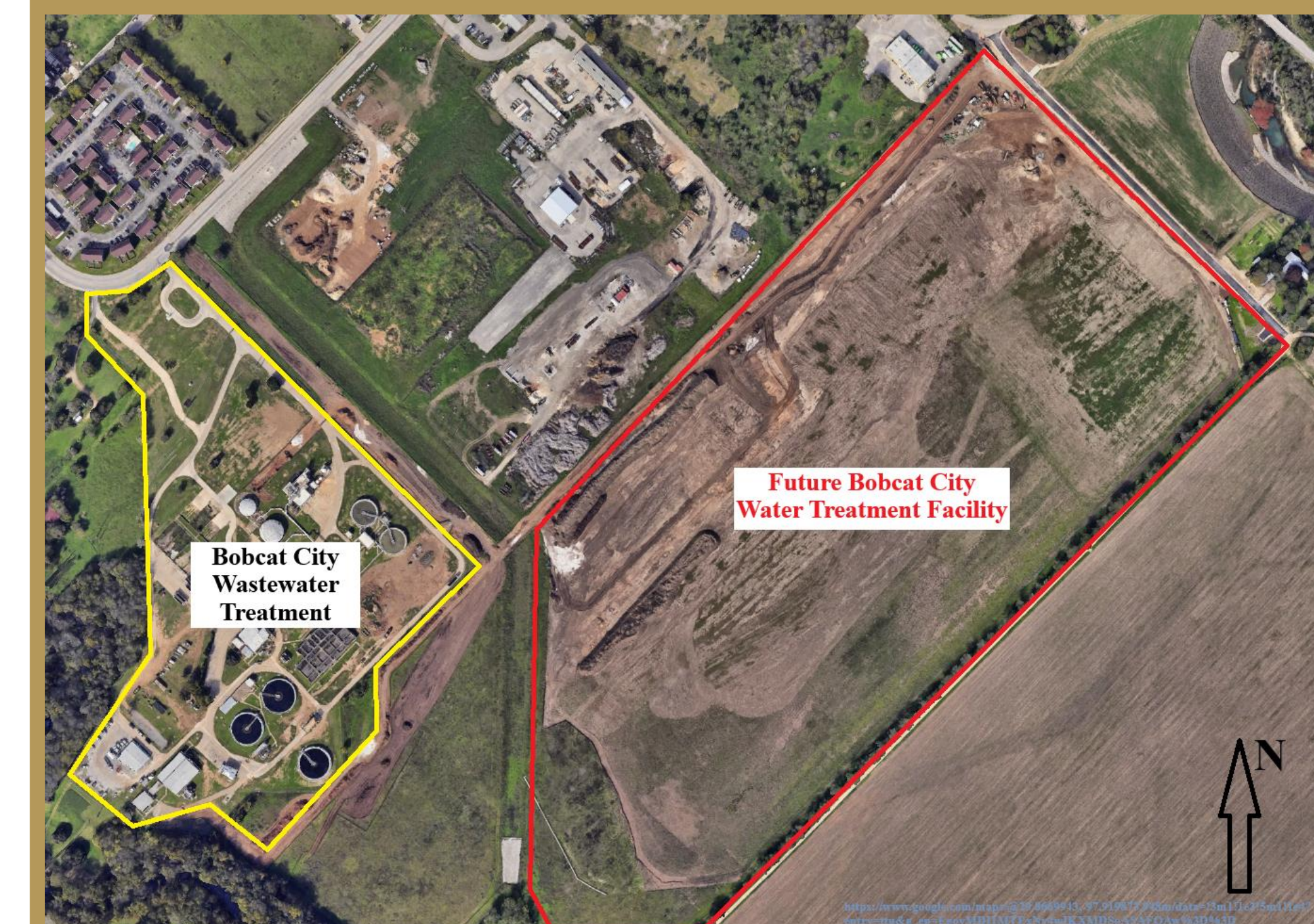
Figure 4: Bobcat City’s Future Water Treatment Location
