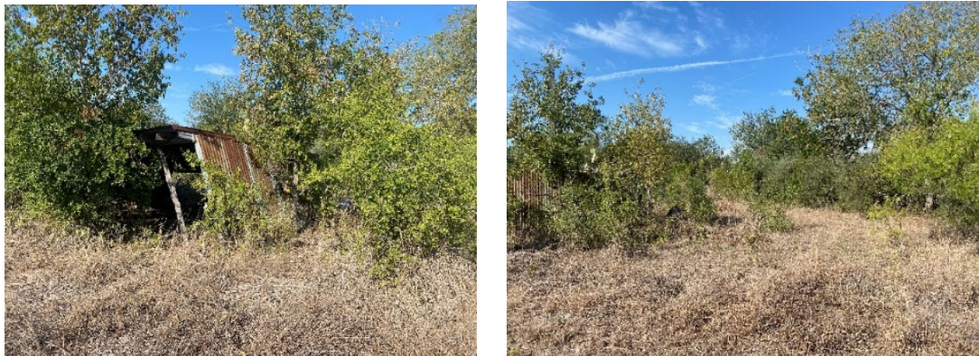
Fig. 14 & 15: Existing Shed to be Removed
