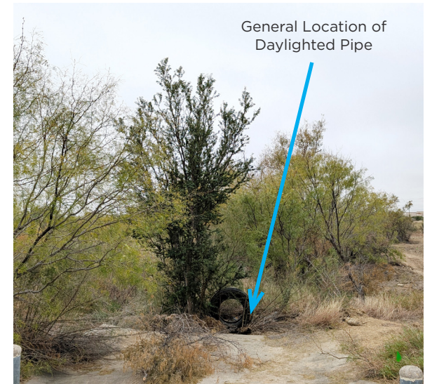
Approximate Location of Daylighted Stormwater Pipe from Medical Drive
