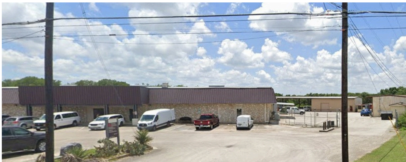
Bobcats Give Back storage location at 1727 Old Ranch Road 12
