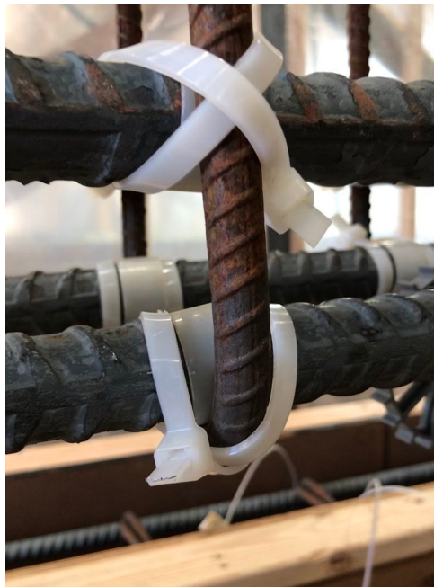
Figure 9. Example of nylon tubing and plastic zip ties used to construct cage. These allowed electrical isolation or inclusion of the different rebars in the ICCP system.
