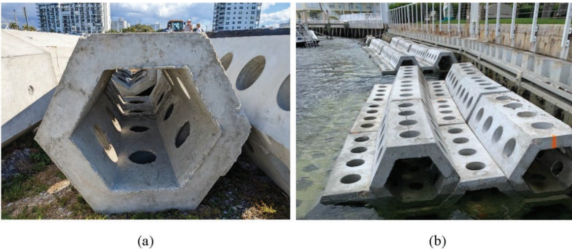
Figure 3. SEAHIVE® elements (a) hexagonal cross section (b) stacked along the coastline.
